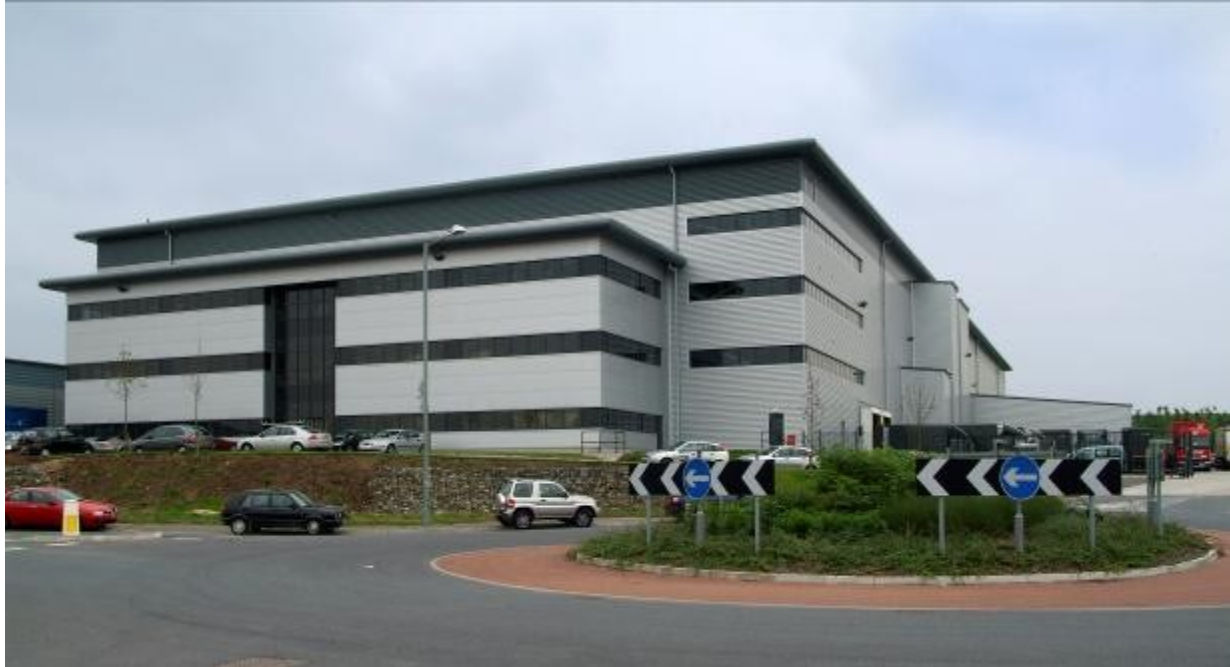
Grahams' new integrated distribution, warehousing and head office site at Matrix Park
